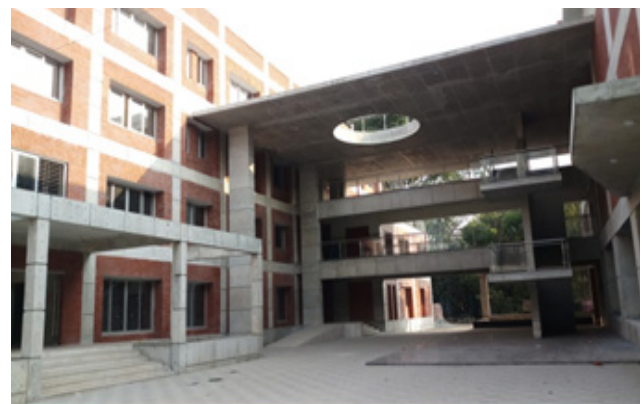
Newly built Foreign Service Academy at State Guest House Sugandha in Baily Road, Dhaka
